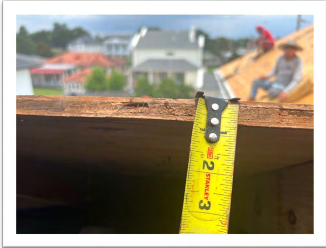
Roof Deck Thickness
