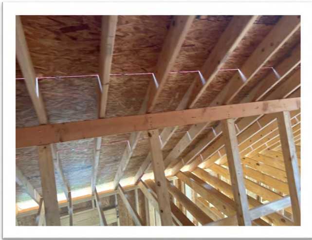
Attic Rafter Photos
