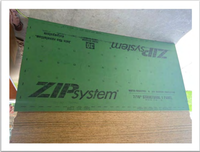
Roof Deck Thickness
