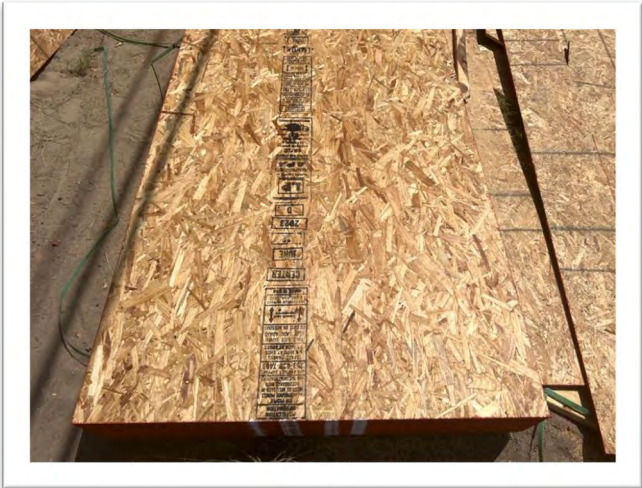
Roof Deck Thickness
