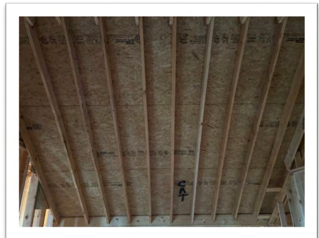
Attic Rafter Photos
