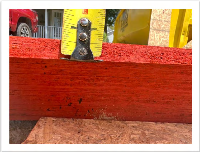
Roof Deck Thickness
