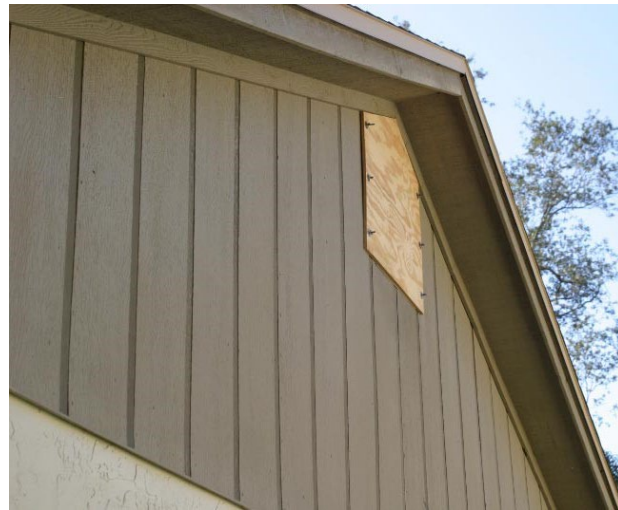
Figure 3.3. Outside shuttering of a gable end vent
