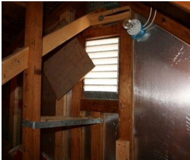
Figure 3.2. Example of a gable end vent with
