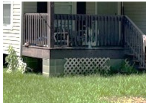
Figure 9. Post and beam/piling
