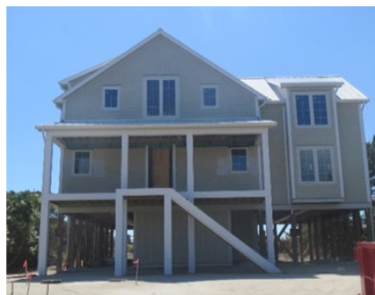
Figure 7. Post and beam/piling
