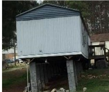
Figure 3. Ineligible dry-stack foundation.
