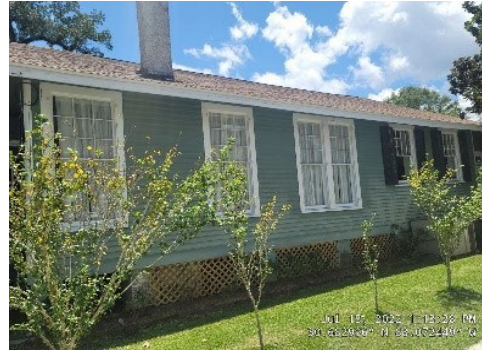
Figure 8. Post and beam/piling.
